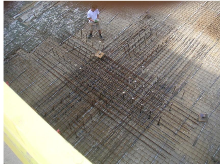
Radier –armature anti-poinçonnement
