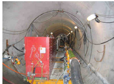
Step down transformer
