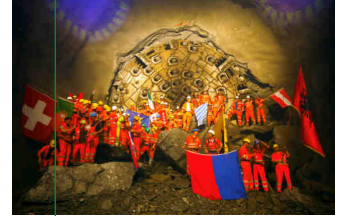
S-210/211 Gotthard Tunnel
