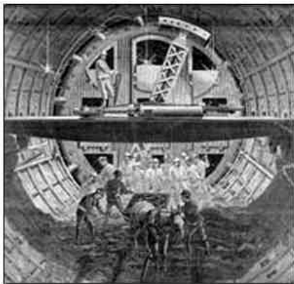
Shields for digging of the metro in Paris 19-20th century (itff)
