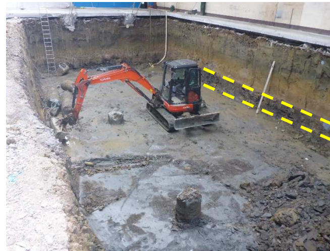
Halle usine Aubange
