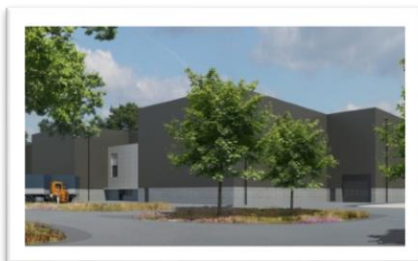
Installation for the Production of Monoliths (IPM)
